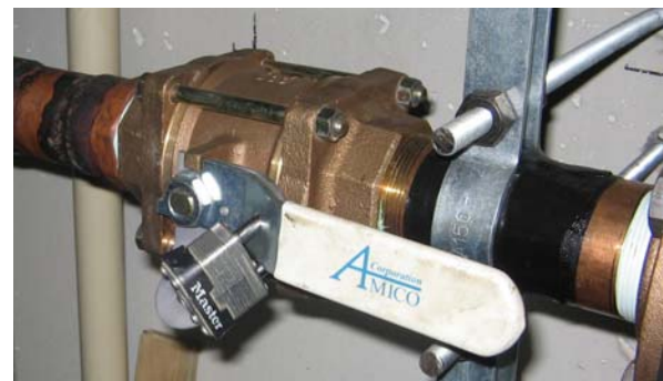
With JRA Plate Installed
